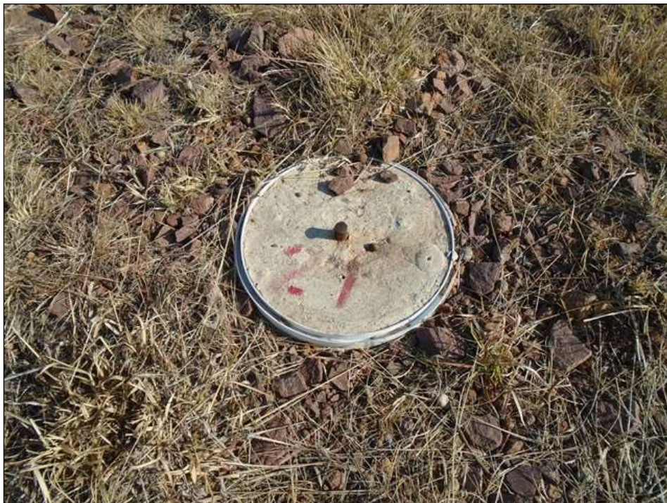
Figure 2: Settlement beacon typical example
