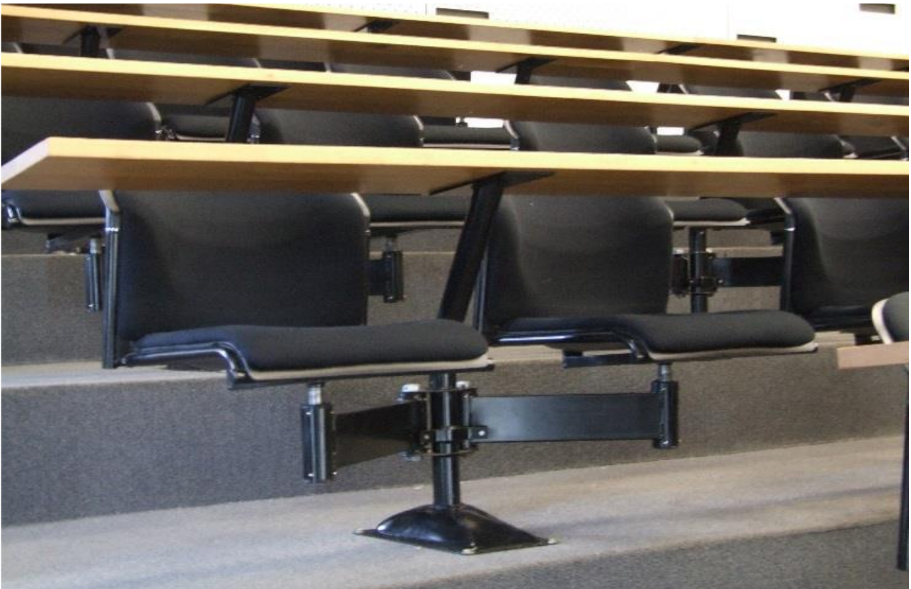
Figure 4.2 Double swing arm mechanism is black epoxy powder coated
