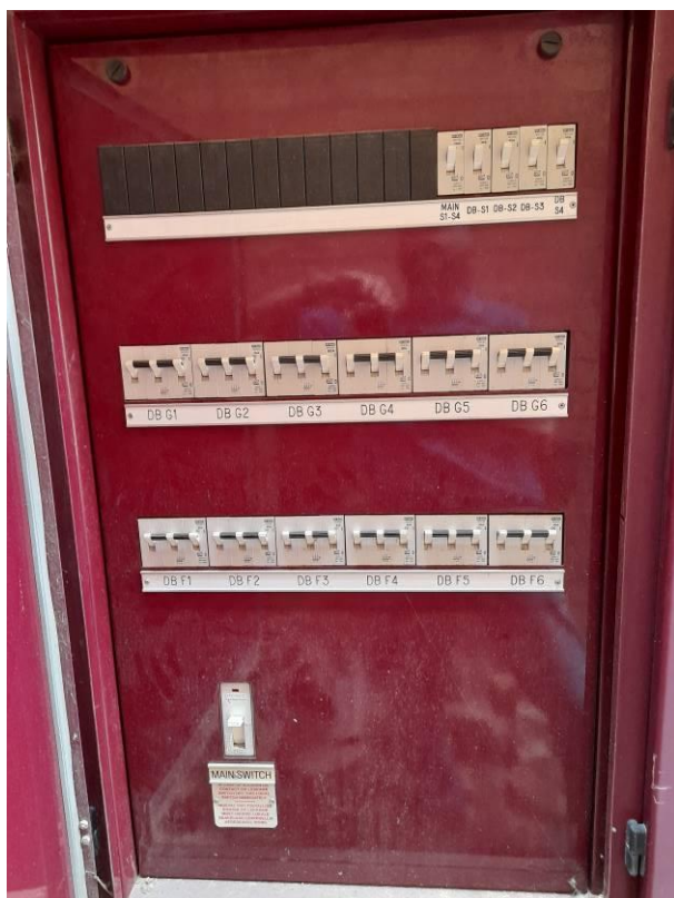
Photo 4 Main Distribution Board: DB – MAIN (DM – M)
