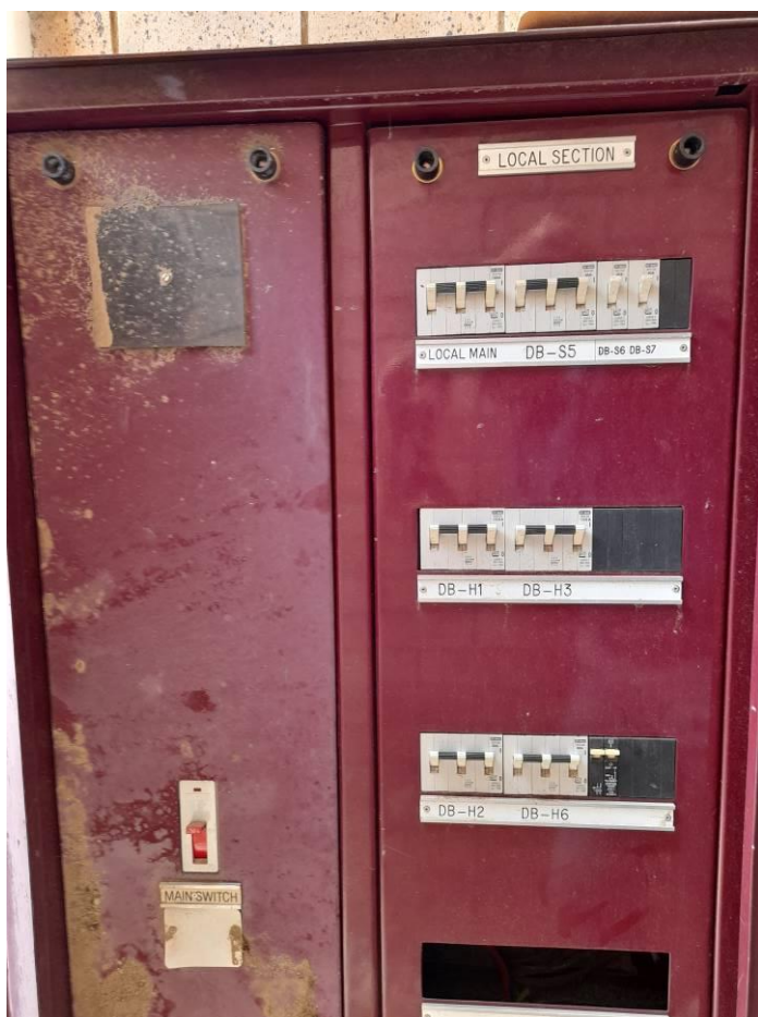
Photo 8 Sub-Main Distribution Board: DB – M1
