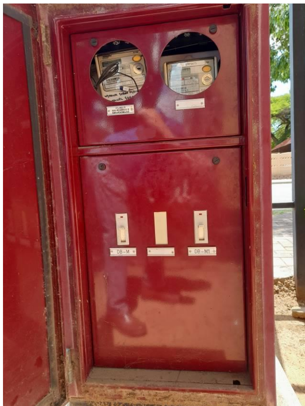
Photo 3 Main Distribution Board at Municipal Connection
