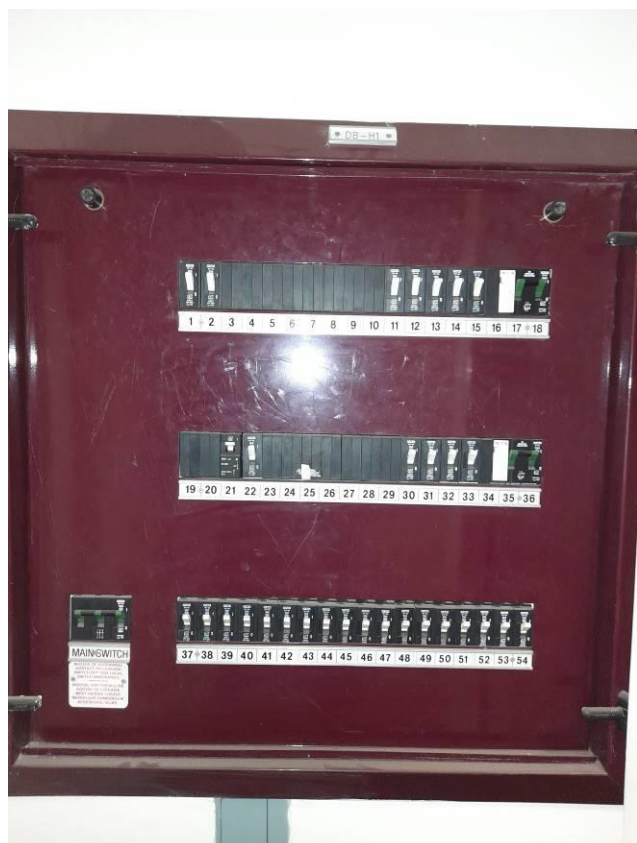
Photo 12 Distribution Board: DB – H1 (DB – G5)
